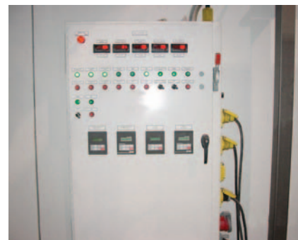
A central control panel in the test lab monitors and controls the equipment operation during testing and toll processing.
